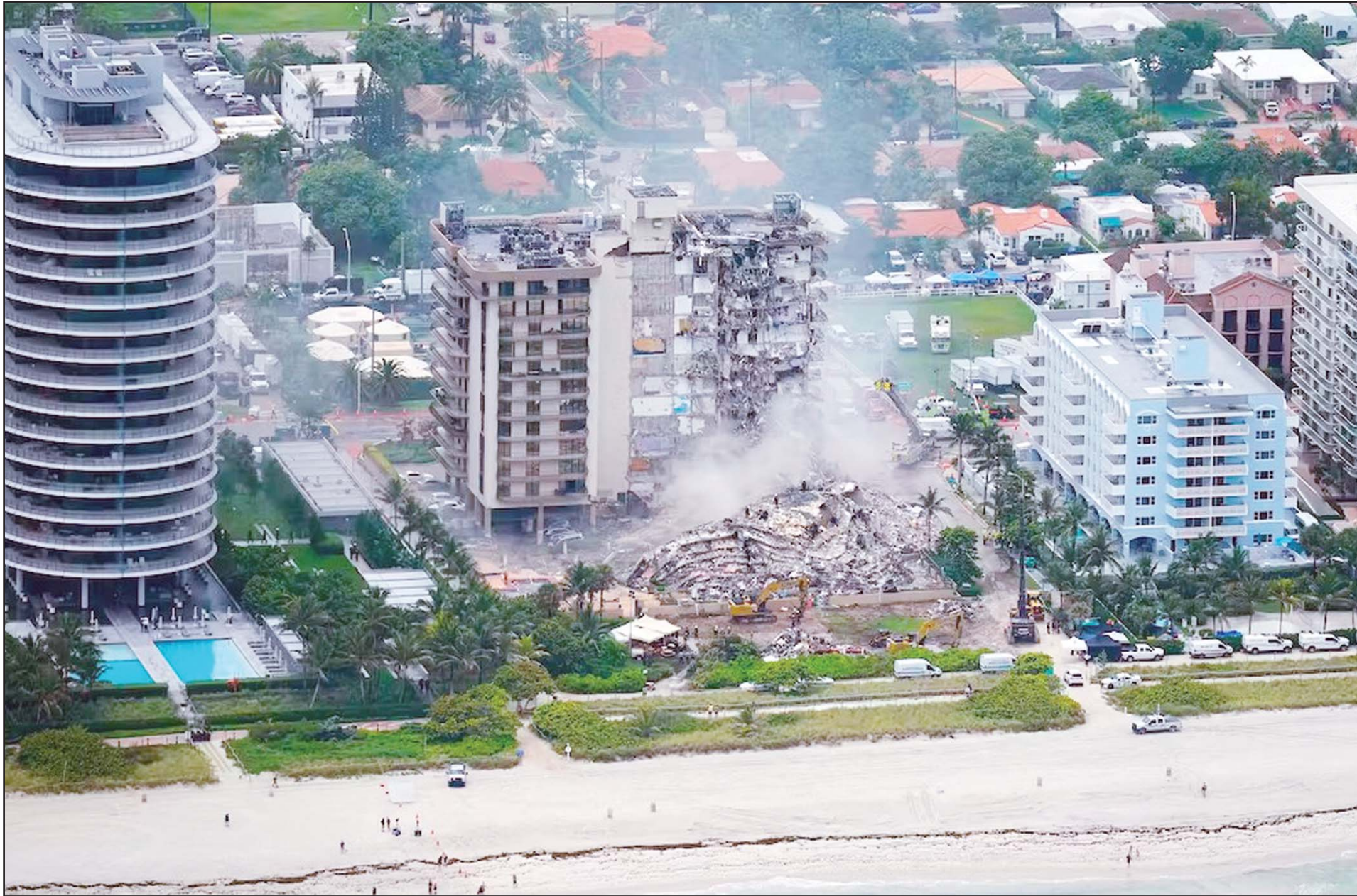
An aerial photo of four condo towers on the beach. In the center is Champlain Towers South, which partially collapsed in June 2021. (AP)
