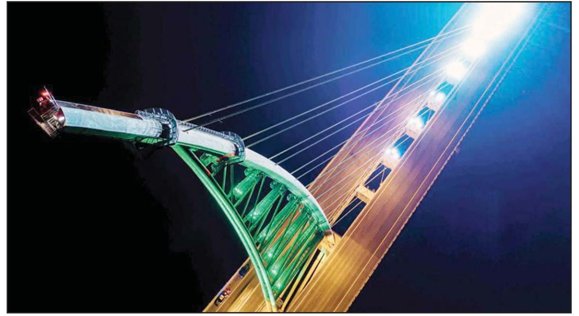
View of Sheikh Jaber Al-Ahmad Bridge.
