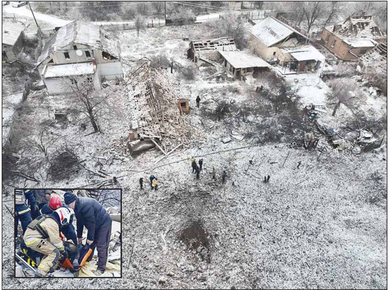
In this photo provided by the Ukrainian Emergency Service, a view of private houses damaged by a Russian missile attack in Novomoskovsk near Kryvyi Rih, Ukraine, Monday, Jan. 8, 2024. Inset: Rescuers help a wounded person after residential houses were destroyed by a Russian missile attack. (AP)
