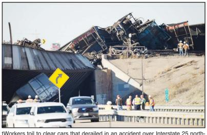
tWorkers toil to clear cars that derailed in an accident over Interstate 25 northbound on Oct 16 north of Pueblo, Colo. A broken rail caused a train derailment that collapsed a bridge over an interstate highway in Colorado, killing a truck driver and blocking the road for days, federal authorities said Tuesday based on their preliminary findings.
