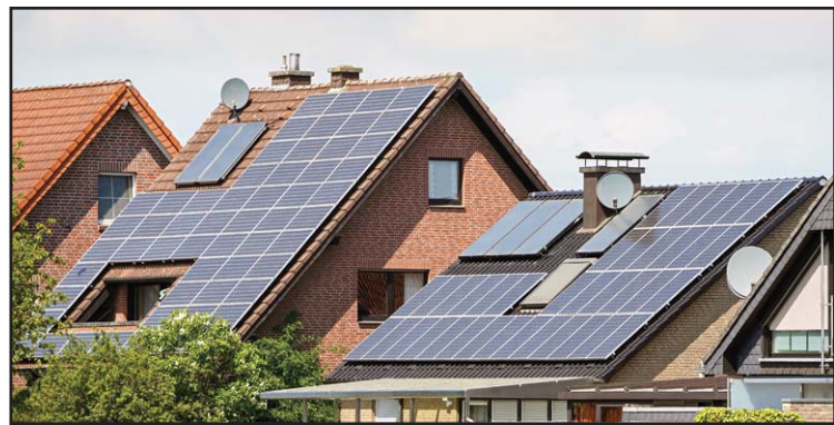
Rooftops on private houses are covered by solar panels to produce renewable electricity in Duellmen, Germany, Tuesday, May 3, 2022. The world is set to add a record amount of renewable electricity capacity this year as governments and consumers seek to offset high energy prices and take advantage of a boom in solar power. (AP)
