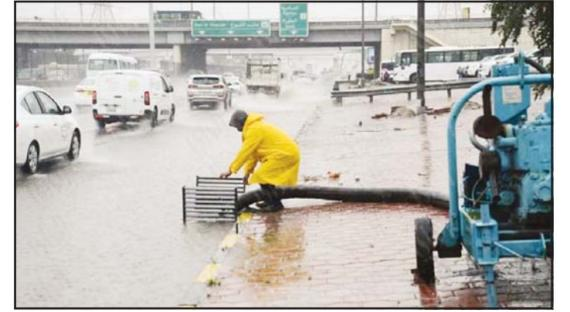
A municipality worker fixes a suction pump to drain rain water from the road.
