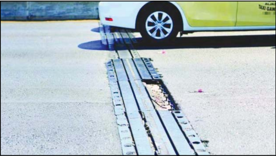
Worn out bridge joints pose risk to motorists.
