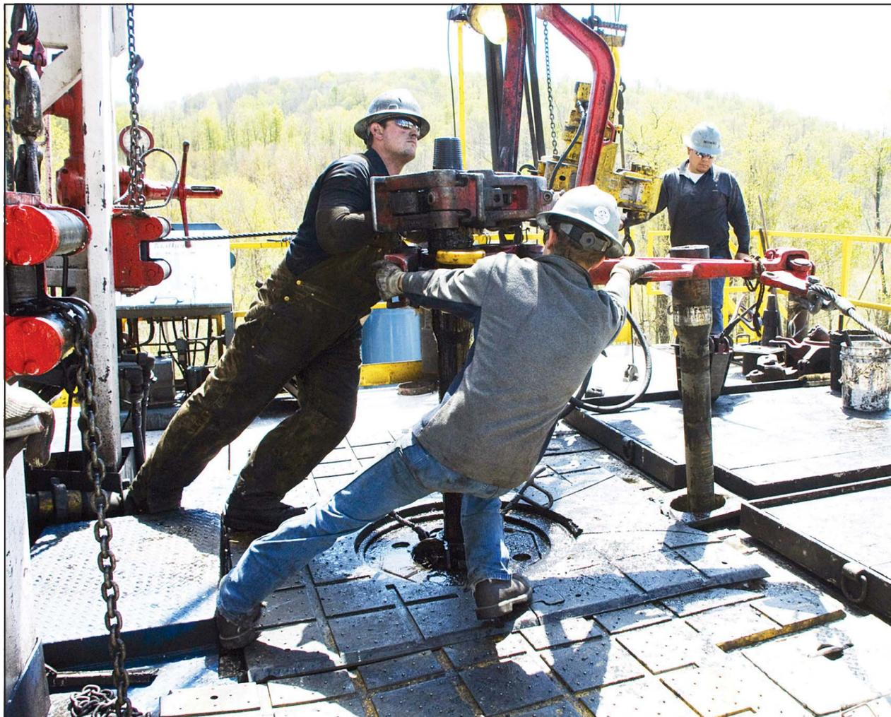
Workers move a section of well casing into place at a Chesapeake Energy natural gas well site near Burlington, Pa., in Bradford County, on April 23, 2010. A team of that has spent four years studying the health effects of natural gas fracking in southwestern Pennsylvania is set to present its findings Tuesday, Aug. 15. (AP)
