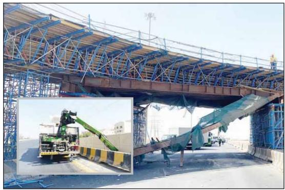
Photos by Rizk Taufiq The iron column that fell from the bridge. (Inset) the truck involved in the accident.
