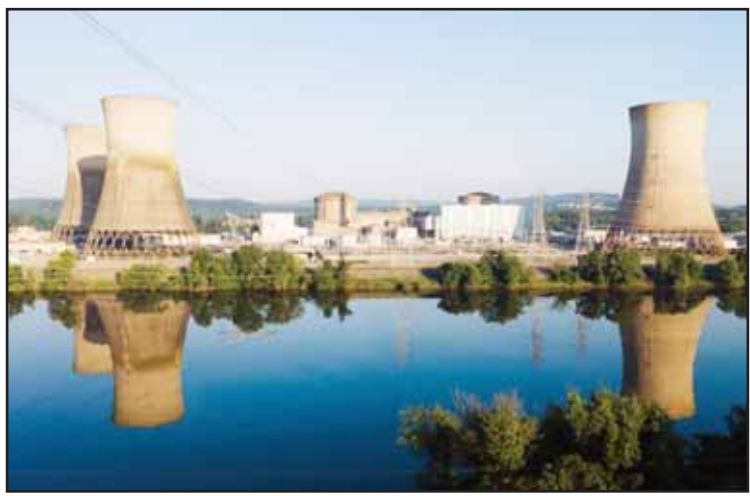
At Constellation’s nuclear power plant on Three Mile Island, called the Crane Clean Energy Center, near Middletown, Pa., the cooling towers are reflected in the Susquehanna River, June 25, 2025. (AP)
