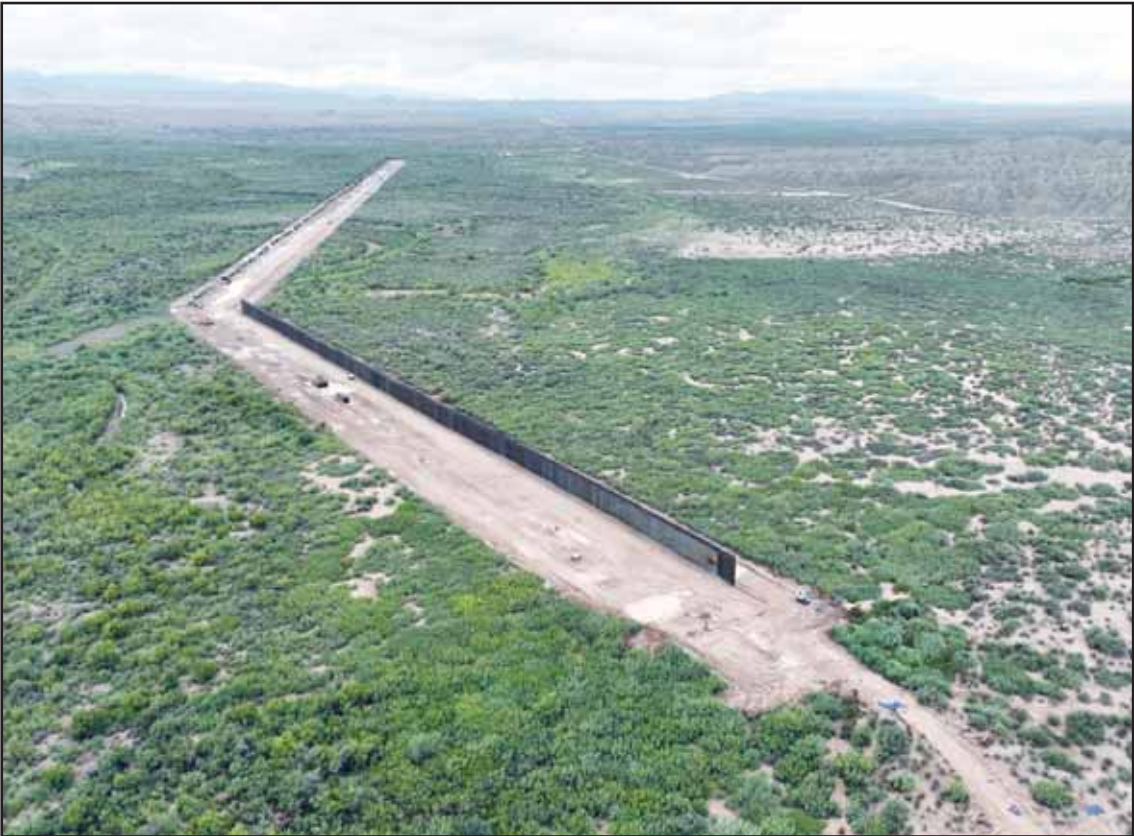
A portion of border wall is under construction in the Big Bend region on Sept 23, near Sierra Blanca, Texas. (AP)
