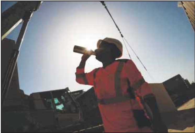
A worker drinks water on a construction site during high temperatures in Boulogne Billancourt, outside Paris on June 24. (AP)
