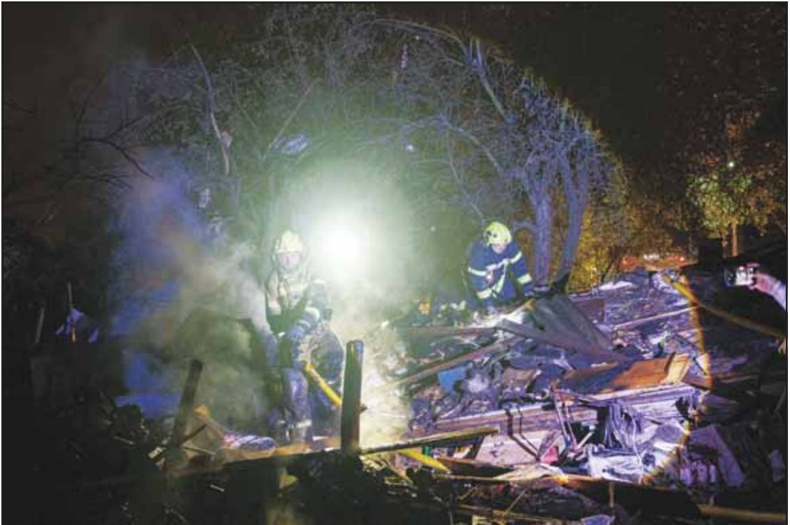
Rescue workers put out a fire at a residential house destroyed in a Russian missile strike on Kyiv, Ukraine on Oct 21. (AP)
