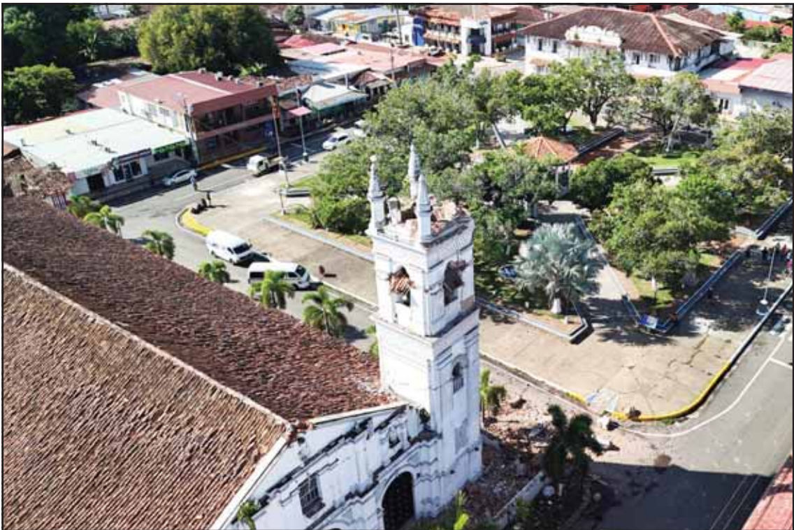
A church tower is damaged after an earthquake struck Villa de los Santos, Panama on Oct 10. (AP)
