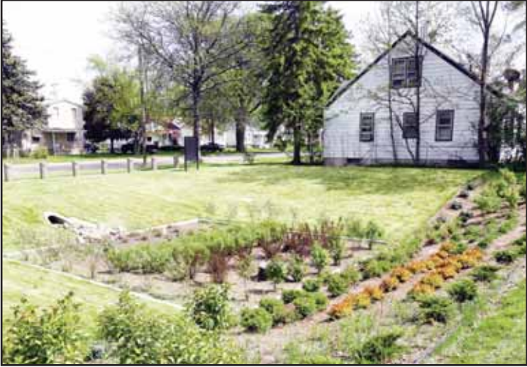
A bioretention garden built to collect rain runoff appears at a home in the Warrendale neighborhood of Detroit on May 16, 2016. (AP)
