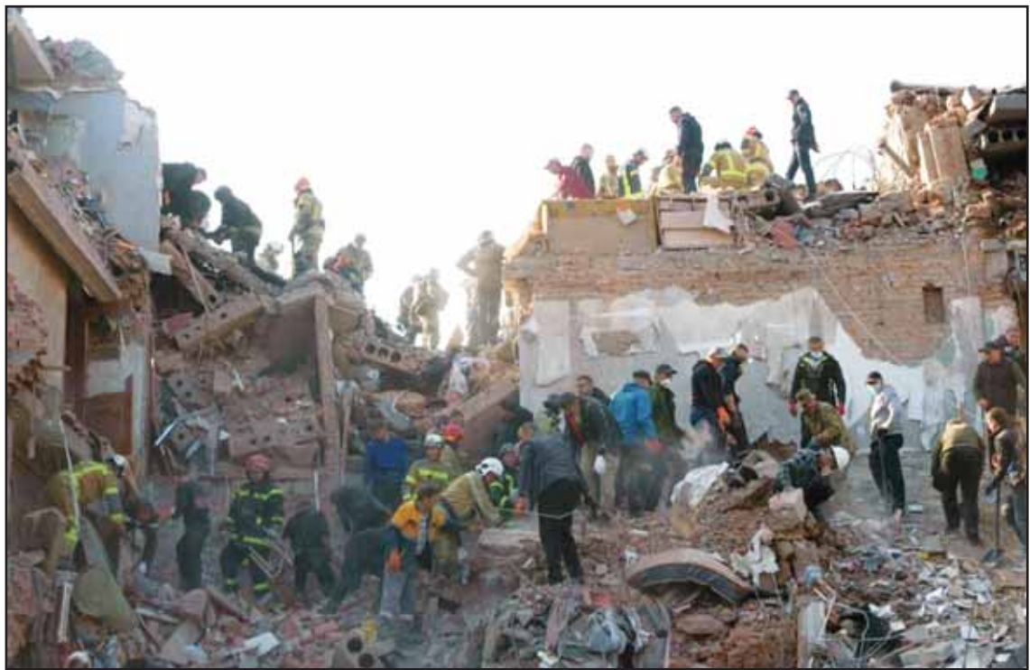
Locals and rescuers clear the rubble of a residential building destroyed in a Russian missile strike on Pryluky, Ukraine on Oct 7. (AP)
