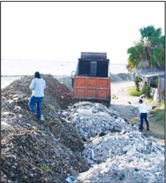
Workers build a barricade to help keep water out of their town as Hurricane Polo approaches in Puerto San Carlos, Baja California Sur state, Mexico on Sept 27. (AP)
