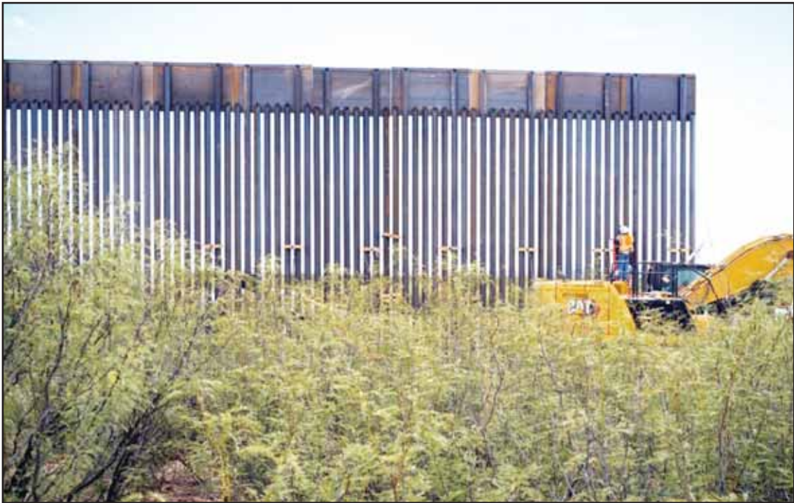
In this photo provided by Scott McWilliams, crews install the first sections of a new border wall in the Big Bend region of west Texas, on Sept 16. (AP)
