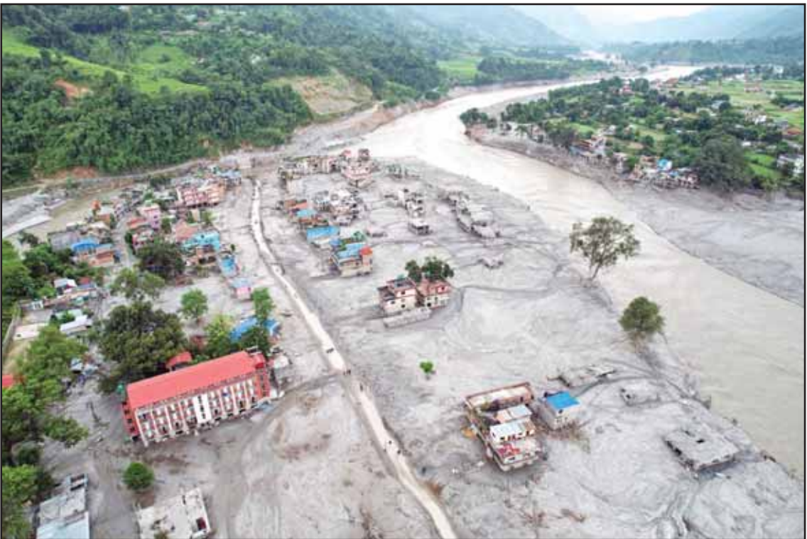
Homes are engulfed in mud in the aftermath of flash flooding along the Trishuli River in the Devighat area of Nuwakot district, Nepal, Aug 29. (AP)
