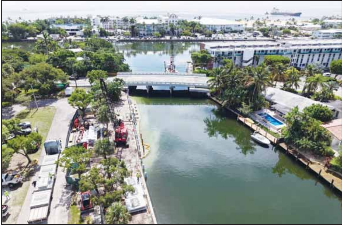
Workers install a 3D-printed living seawall manufactured by Kind Designs at the Church by the Sea on Aug 4, in Fort Lauderdale, Fla. (AP)
