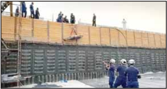
Rescue operation in progress.
