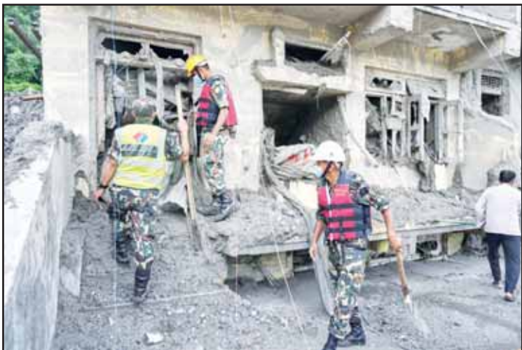
Rescuers inspect a residential building damaged in the aftermath of the flash floods in Nepal's Nuwakot district on Sept. 2. (AP)
