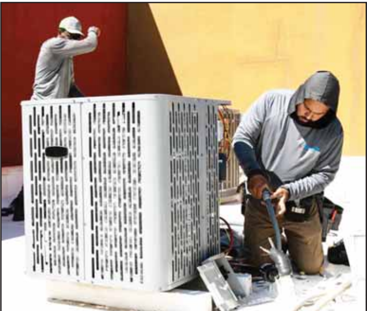
Sonel Telemaque, (left), wipes sweat from his brow while installing a new air conditioning unit alongside Brian Hermosillo during record-breaking heat, March 19 in Tempe, Ariz. (AP)
