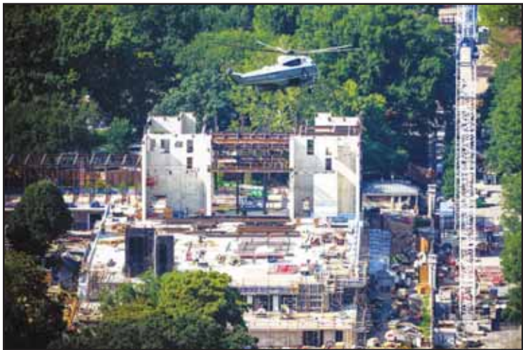
Marine One with President Donald Trump passes over construction on the new White House ballroom on Aug 21, seen from the Washington Monument in Washington. (AP)
