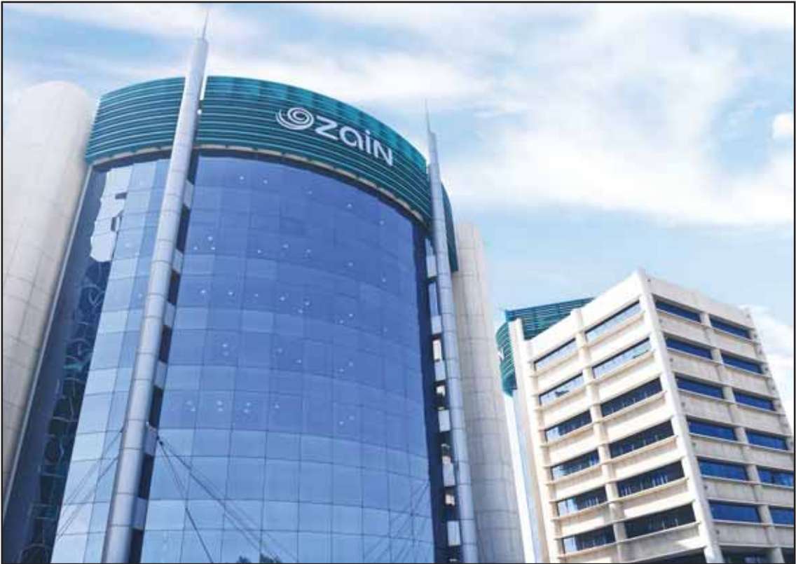
Zain Group HQ building
