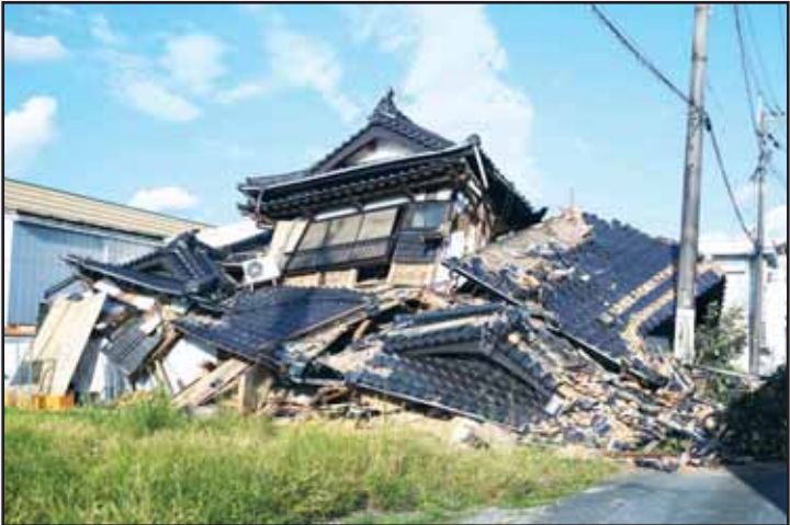
A collapsed building is seen in Yatsushiro, southwestern Japan on July 29, the day after an earthquake hit the area. (AP)
