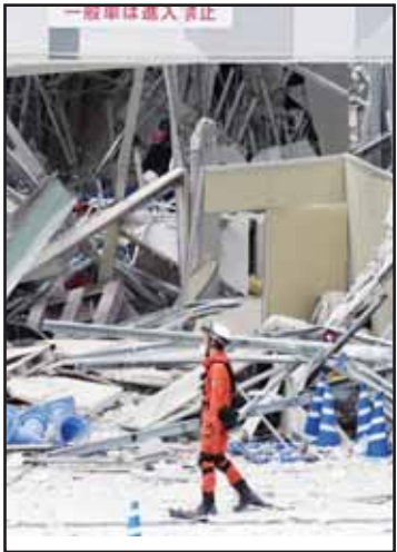
A rescue worker walks in front of Aeon Mall, which was damaged by an explosion following an earthquake, is seen in Kashima, Kumamoto Prefecture, southern Japan on July 29. (AP)
