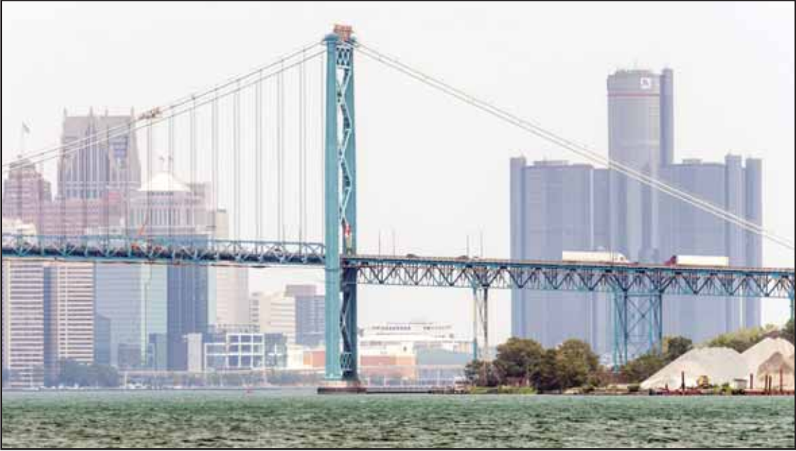
Transport trucks are seen using the Ambassador Bridge on the first day of opening for the Gordie Howe International Bridge, in Windsor, Ontario on July 27. (AP)
