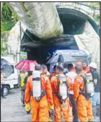
Members of the rescue team carry oxygen cylinders outside the entrance to an under-construction tunnel at a hydropower project in Samardung village, about 40 kilometers (25 miles) from Gangtok, India on July 21. (AP)
