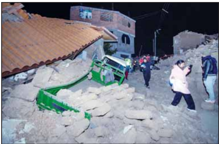
Residents walk amid the debris of homes that collapsed after an earthquake struck Pumpuya, Peru on July 19. (AP)
