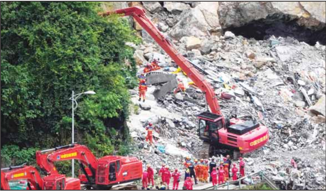
Rescuers use a heavy duty machine to clear the rubble to search for trapped victims at the scene of a landslide in Pengshui County in southwestern China's Chongqing on July 18. (AP)
