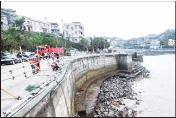
Steel frames are installed along a road where guardrails were blown down by strong winds in Yuhuan of Taizhou City, east China's Zhejiang Province on July 12. (Xinhua)
