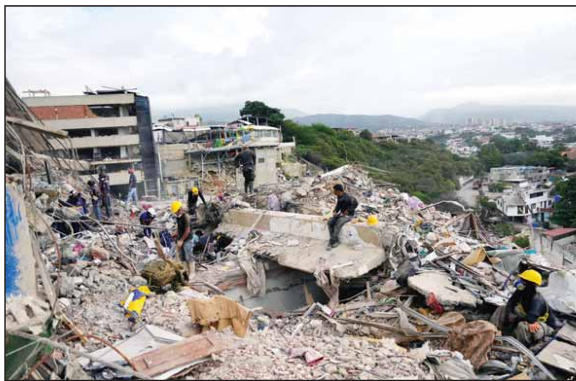
Rescue workers search through the rubble on a building collapsed during the earthquakes in La Guaira, Venezuela on July 6. (AP)
