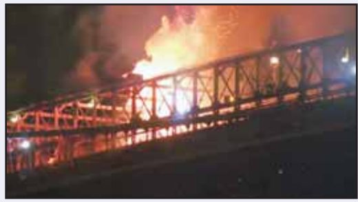
In this image taken from video, a fire breaks out on the Brooklyn Bridge in New York during the city's fireworks celebration on July 4. (AP)
