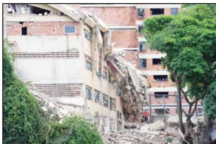
Part of the San Judas Tadeo school collapsed in Caracas, Venezuela, on July 3, days after it was damaged in the earthquakes. (AP)
