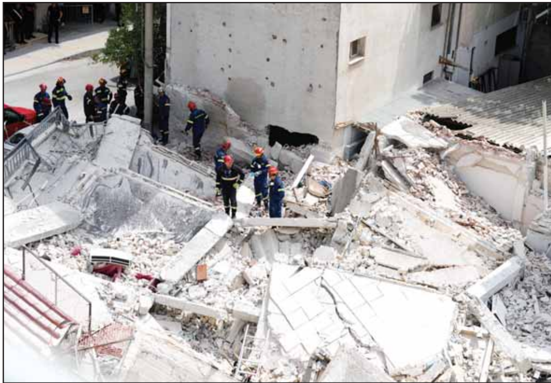
Greek rescue crews search through the rubble of a building that collapsed in the Petralona neighborhood of central Athens on June 30. (AP)
