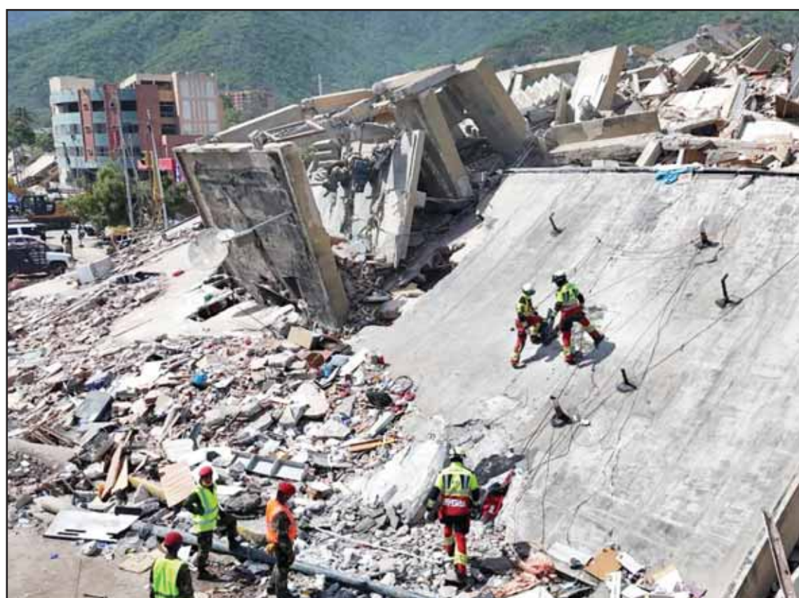
Mexican Army rescue workers search for people trapped in collapsed buildings after earthquakes struck La Guaira, Venezuela on June 28. (AP)
