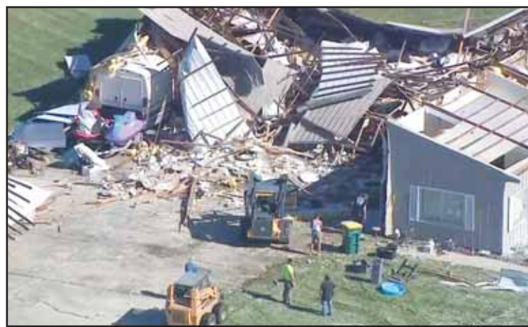
This photo made from video provided by WLS shows an aerial view of storm damage on June 12, in Merrillville, Ind. (AP)
