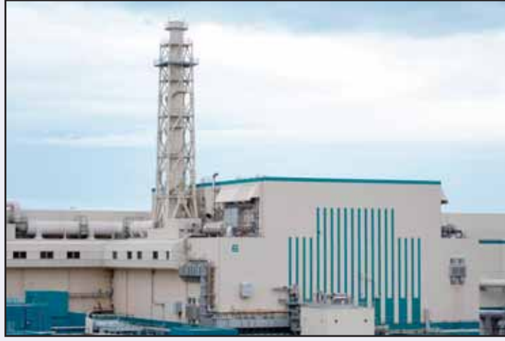
The Unit 6 reactor building is pictured during a media tour at Tokyo Electric Power Company Holdings' (TEPCO) Kashiwazaki-Kariwa nuclear power station in Kariwa Village, Niigata prefecture, Japan on May 1. (AP)
