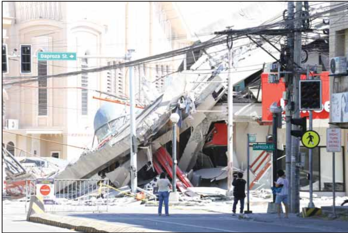
A building is damaged after an earthquake in General Santos, Philippines on June 8. (AP)
