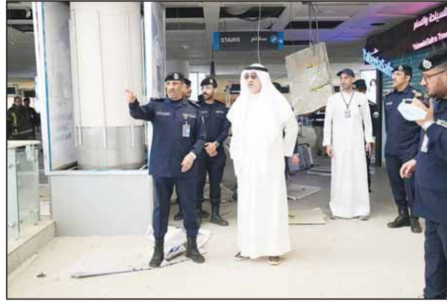
Ministry of Interior photo 1st Deputy Prime Minister and Minister of Interior Sheikh Fahad Yusef Saud Al-Sabah conducts an inspection of Terminal 1, assessing damage and being briefed on the handling of the incident and its aftermath.
