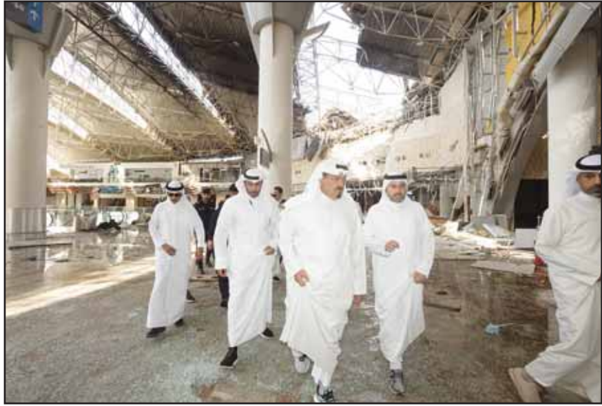
PM Diwan photo His Highness the Prime Minister Sheikh Ahmad Abdullah Al-Ahmad Al-Sabah inspects damage at Terminal One of Kuwait International Airport following the Iranian drone attack, directing immediate repairs and reviewing measures to restore operations.
