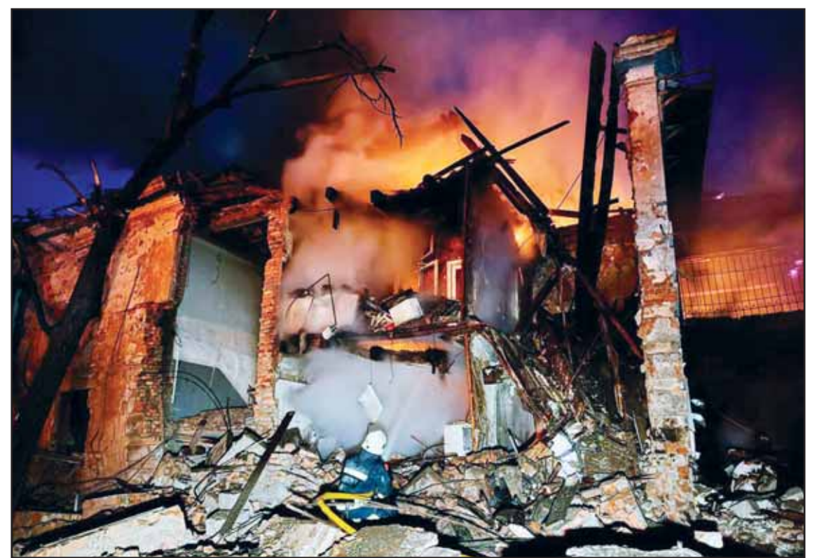
In this photo provided by the Ukrainian Emergency Services on June 2, a rescue worker puts out a fire of a residential building destroyed after a Russian strike on Dnipropetrovsk region, Ukraine. (AP)
