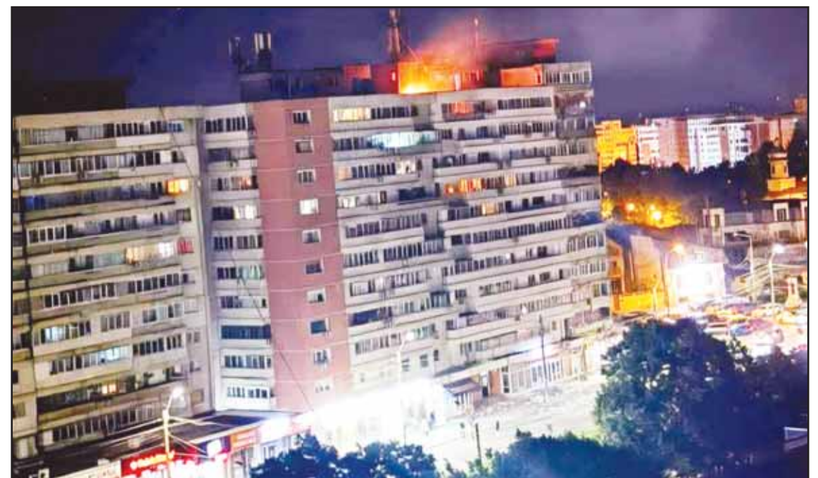
This photo released by Romania's Department for Emergency Situations shows a fire on top of a block of flats after a drone crash caused an explosion and fire on impact, in Galati, eastern Romania near the Ukrainian border on May 29. (AP)
