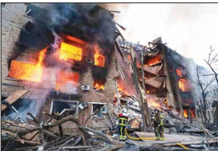
Rescue workers put out a fire of residential building destroyed after a Russian strike in Kyiv, Ukraine, on May 24. (AP)
