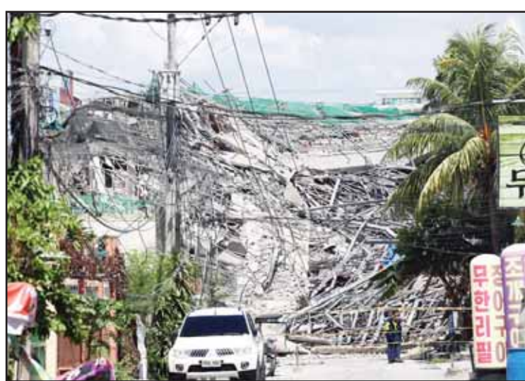
Caution tape marks the area around a collapsed building in Angeles city in Pampanga province, north of Manila, Philippines on May 24. (AP)
