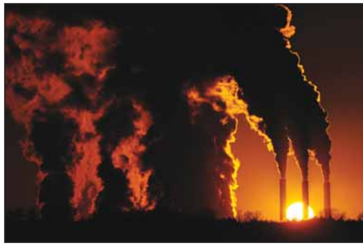
The Jeffrey Energy Center coal-fired power plant operates at sunset near Emmett, Kan on Jan 3, 2026, in Topeka, Kan. (AP)
