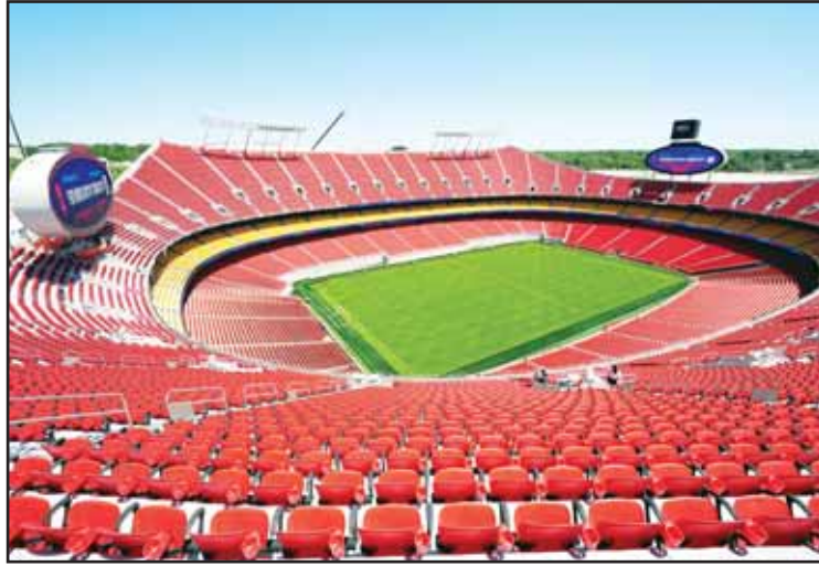
A general view of Arrowhead Stadium as it is rebranded as Kansas City Stadium ahead of the 2026 FIFA World Cup soccer matches in Kansas City, Mo. (AP)
