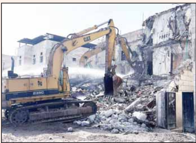
A dilapidated building crumbles under controlled demolition, marking another step in Kuwait's safety drive in Jleeb Al-Shuyoukh. Kuwait Municipality photo
