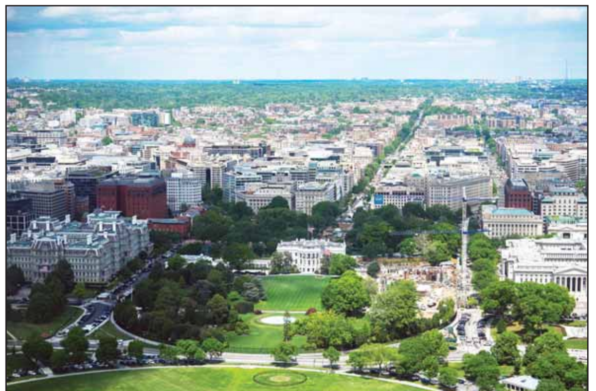
Construction on the new White House ballroom is seen from the Washington Monument, Monday, April 20, 2026, in Washington. (AP)
