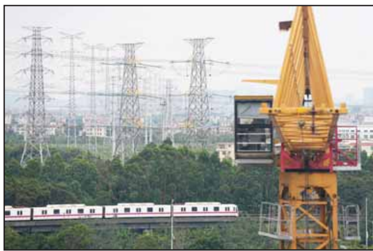
A subway train passes by power lines, in Guangzhou, in southern China's Guangdong province, Thursday, April 16, 2026. (AP)
