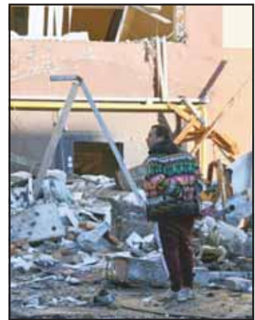
A local man stands in front of a residential building which was heavily damaged after a Russian strike in Odesa, Ukraine on April 6. (AP)
